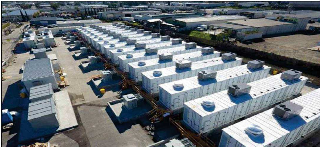
Figure 13: Example of a Lithium-Ion BESS installation
